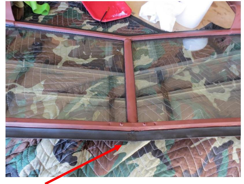
Your thumbs will get sore from working the gasket so expect that. This is one of several ways of installing the gasket.
