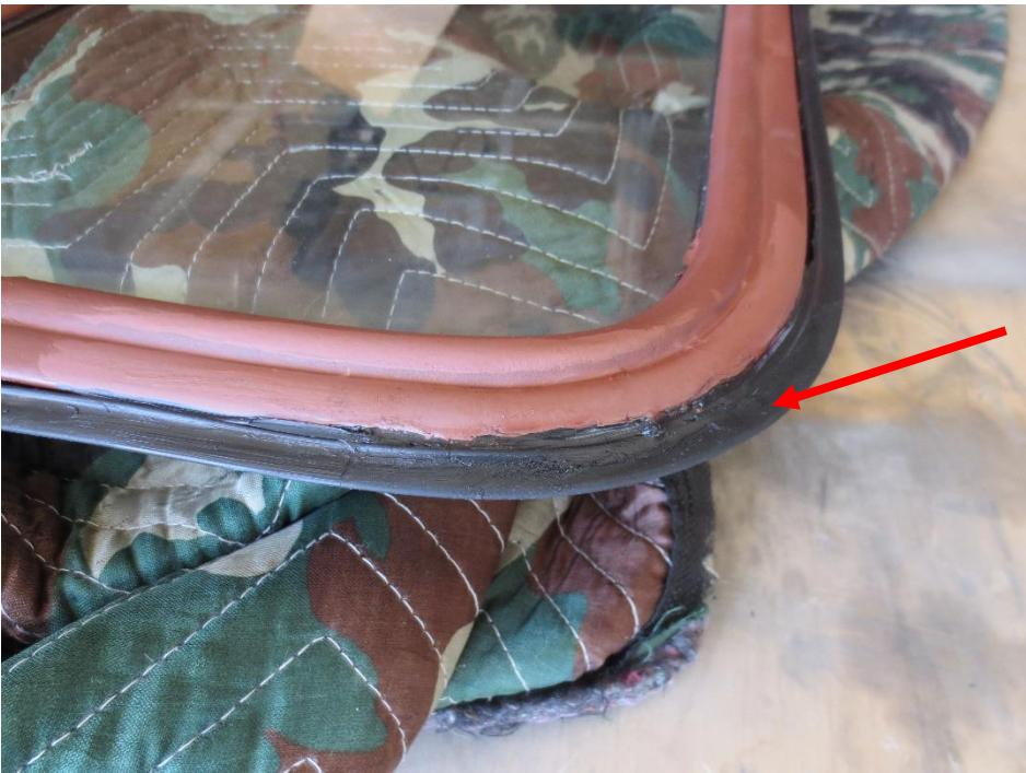
9. If you are installing a non-continuous gasket, you will need to cut off any excess length and fill the gap. RTV Silicone works well to do this.
